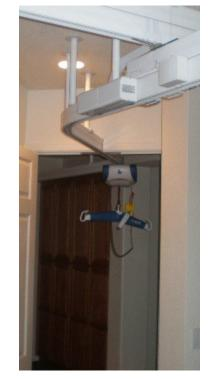
Interlock Gate to transfer from moving XY Track to Fixed Track
